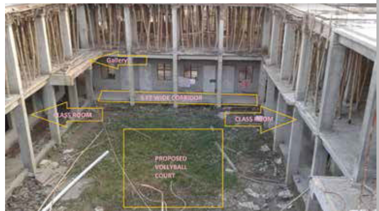
ABOVE: Hope House construction well underway: second storey with courtyard plans
