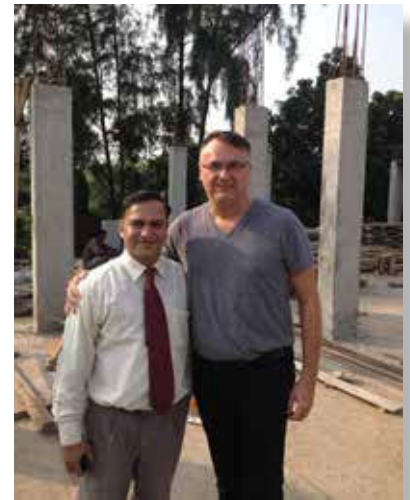
Board member Don Winsor with Pastor Philip at Hope House construction site
